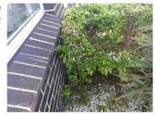
The external vents/weep holes are either covered completely or partly concealed. This can allow concealed termite entry and we recommend that all vents/weep holes be exposed and kept clear of soil, foliage, debris, stored items or other obstructions.
