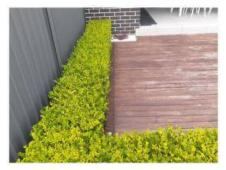
Trees, tree roots, vines or shrubs are close to or abutting the external walls of the structure. This can allow concealed termite entry and they should be removed.
