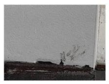
Shrinkage cracks are evident to rendered wall areas. This cracking generally occurs during the curing process of construction. Cracking of this type is an appearance defect and is not considered to be of a structural nature. Some repairs may be required prior to next painting to provide a suitable finish.
