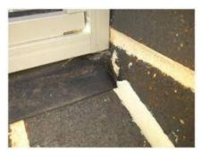
Storm moulds are not present and need to be fitted to ensure water does not penetrate wall cavity. Rectification is required.
