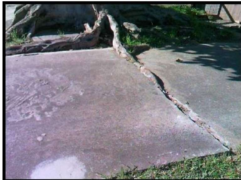
Structural Defect Cracking: Crack Type: Differential movement cracking Width: 15mm Length: 3.0M.
