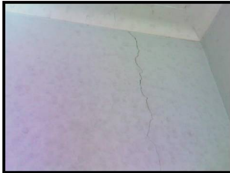
Structural Defect Cracking: Crack Type: Differential movement cracking Width: 15mm Length: 3.0M.
