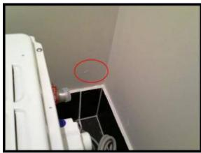
Painting to the vanity side wall is not complete, appears transparent and requires rectification to provide a suitable finish.
